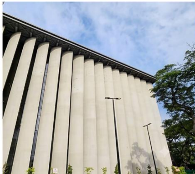
Picture 3: 32m aerofoil shaped reinforced concrete. Photo credits: Meinhardt (Singapore) Pte Ltd
