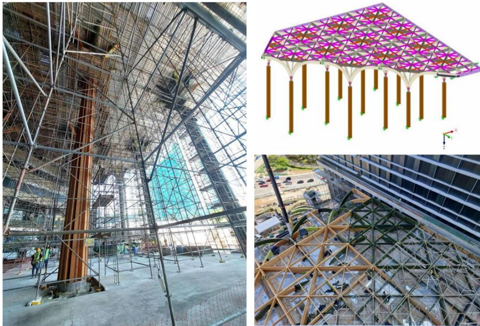
Picture 8: Analysis model and construction of Singapore's tallest arched MET canopy structure. Photo credits: CapitaLand, Ronnie and Koh Consultants Pte Ltd
